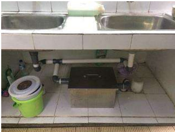
Grease trap Limbah Air Cuci Kantin (Air)
