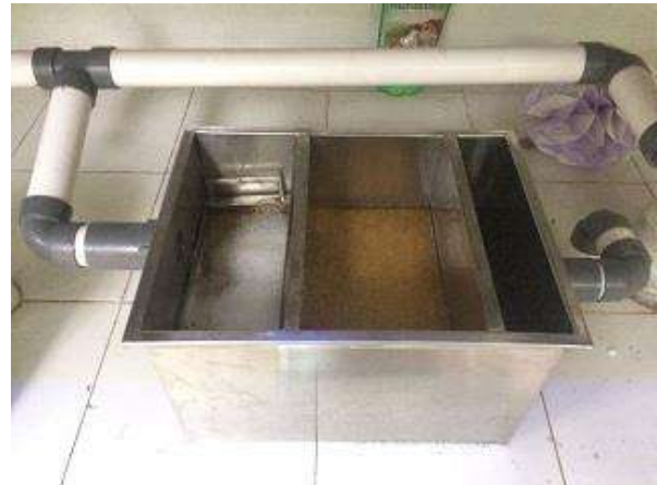
Grease trap Limbah Air Cuci Kantin (Air)
