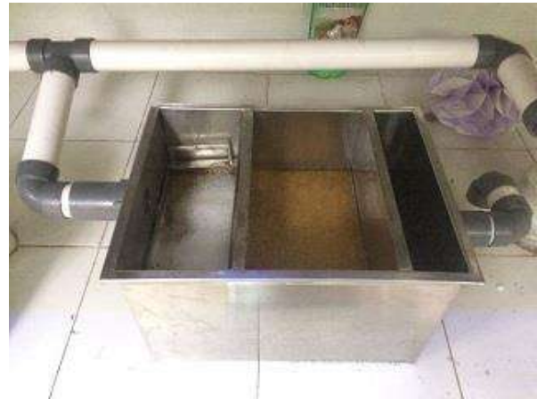
Grease trap Limbah Air Cuci Kantin (Air)
