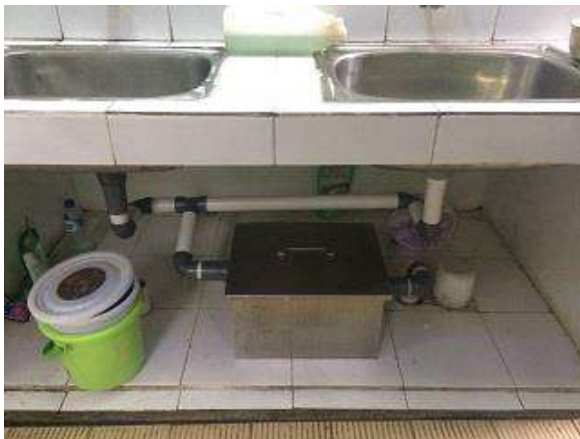
Grease trap Limbah Air Cuci Kantin (Air)
