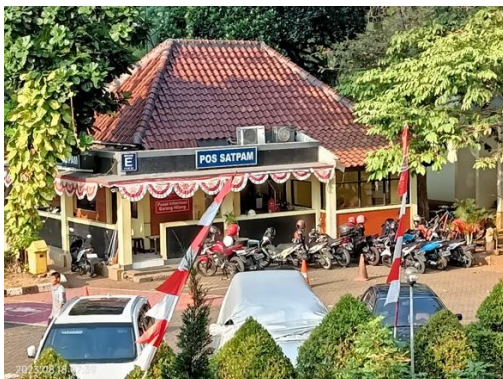
Gedung E FKM UI (Pos Satpam)
