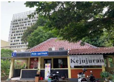
Gedung E FKM UI (Pos Satpam) (Area: 499 m 2 )
